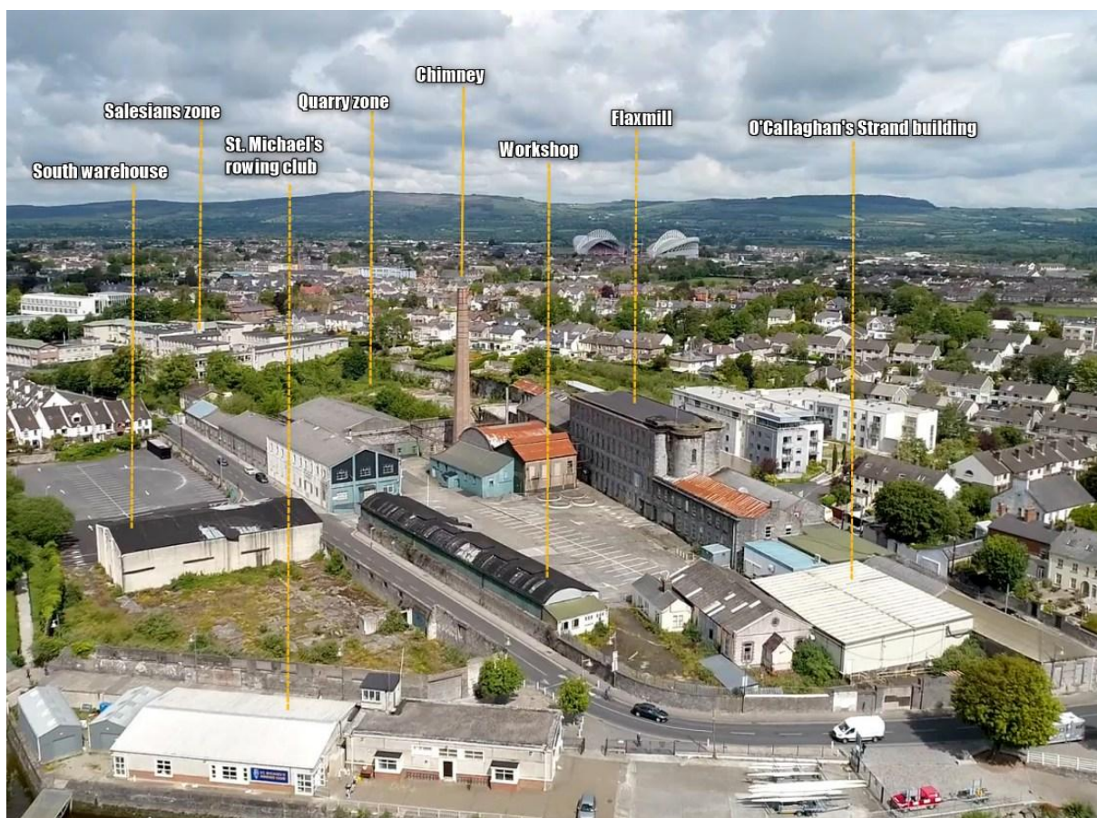
Figure 12.6: Aerial view of the existing subject site looking north-west.
