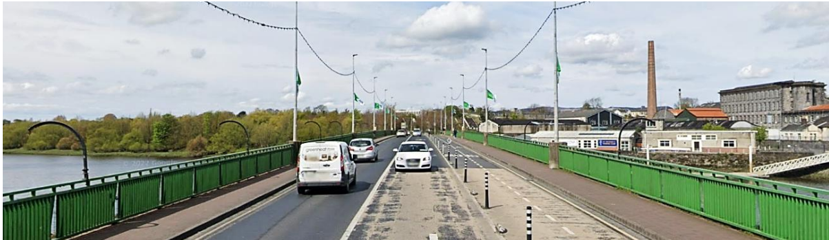
Figure 12.8: Existing view north-westwards along Shannon Bridge. The site is on the right.
